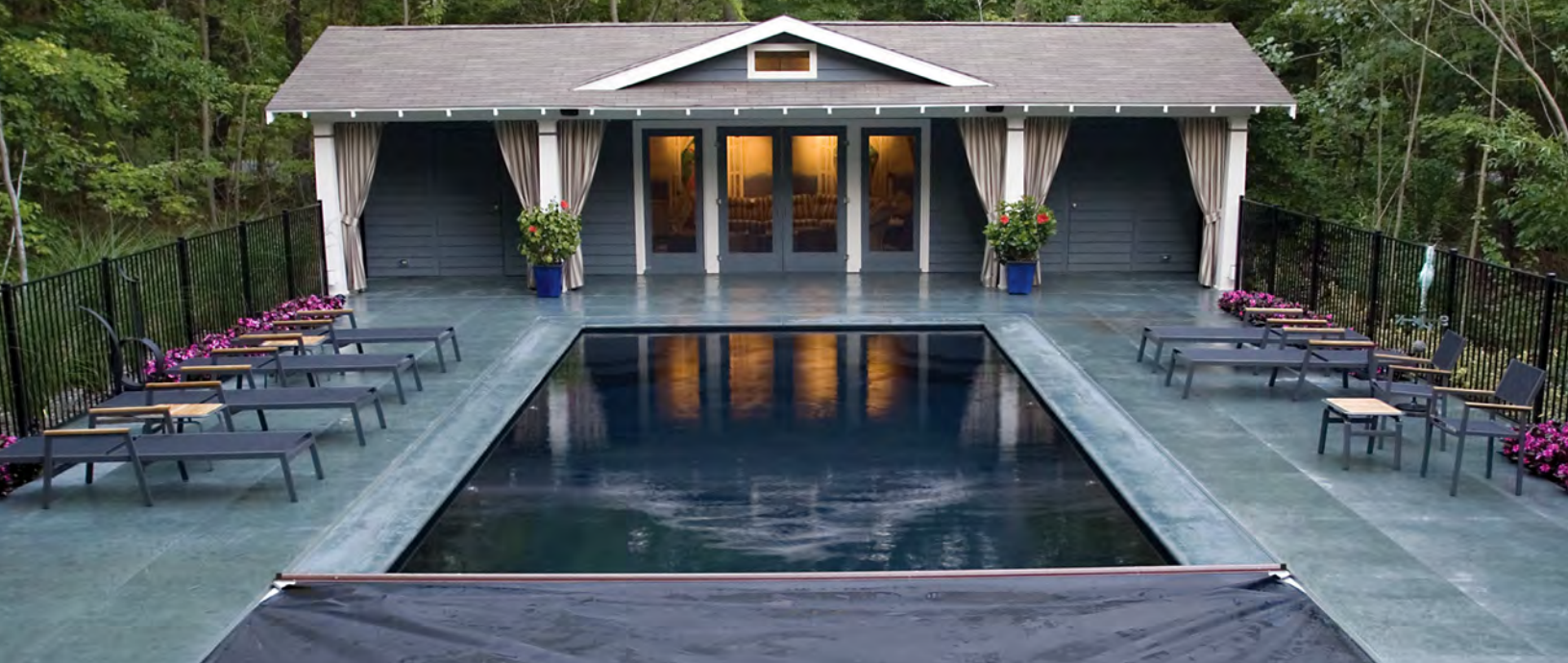
Perimeter overflow pool
